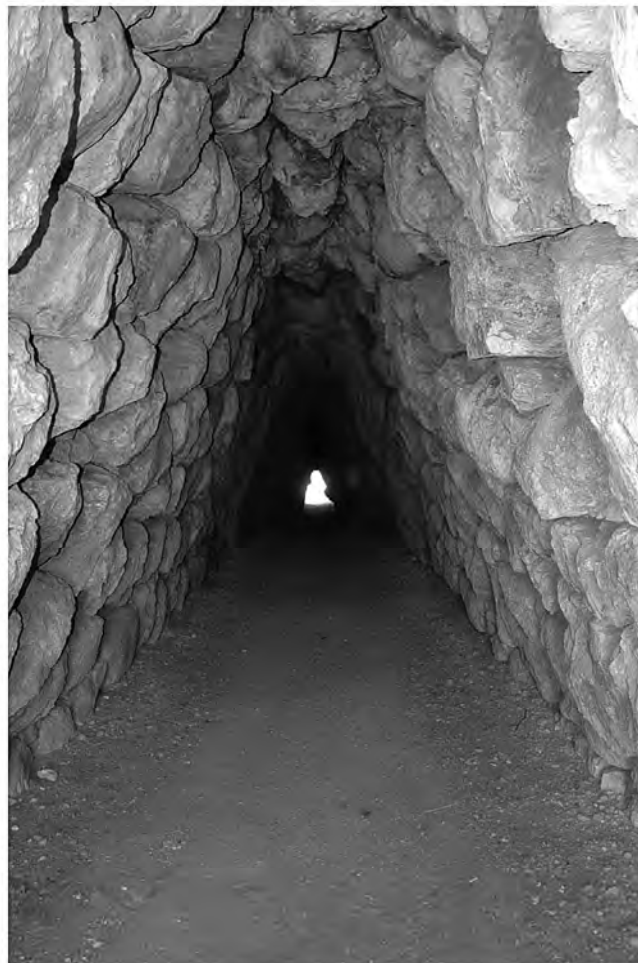
Figure 6: Photo of the two-dimensional arc inside the walls at Hattuša with very rough stone fitting
