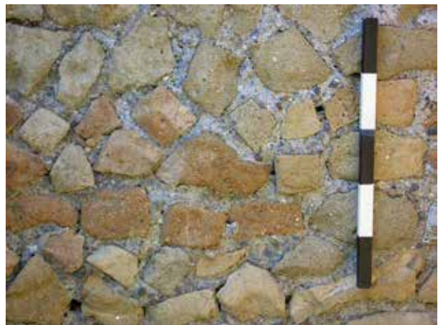
Figure 11.3d: Horrea, via degli Aurighi (III.ii.6). Rubble facing of dividing walls (photo: Janet DeLaine).
