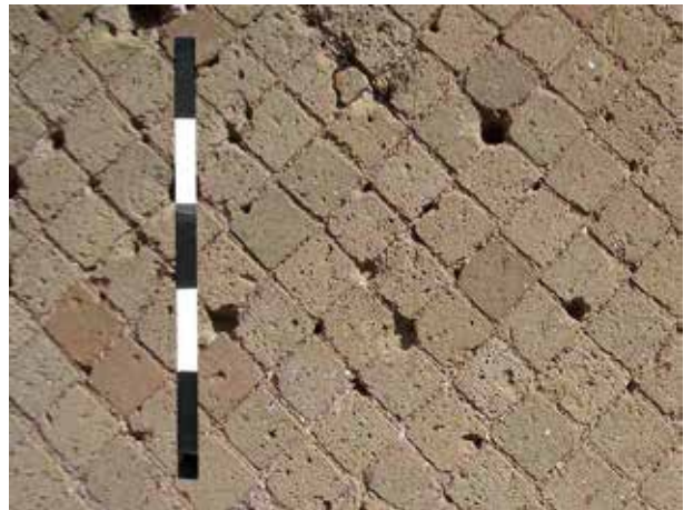
Figure 11.3b: Horrea, via degli Aurighi (III.ii.6). Fine reticulate of façade (photo: Janet DeLaine).
