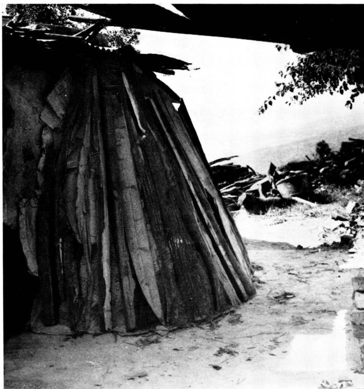
B. Main loading door blocked for firing.
