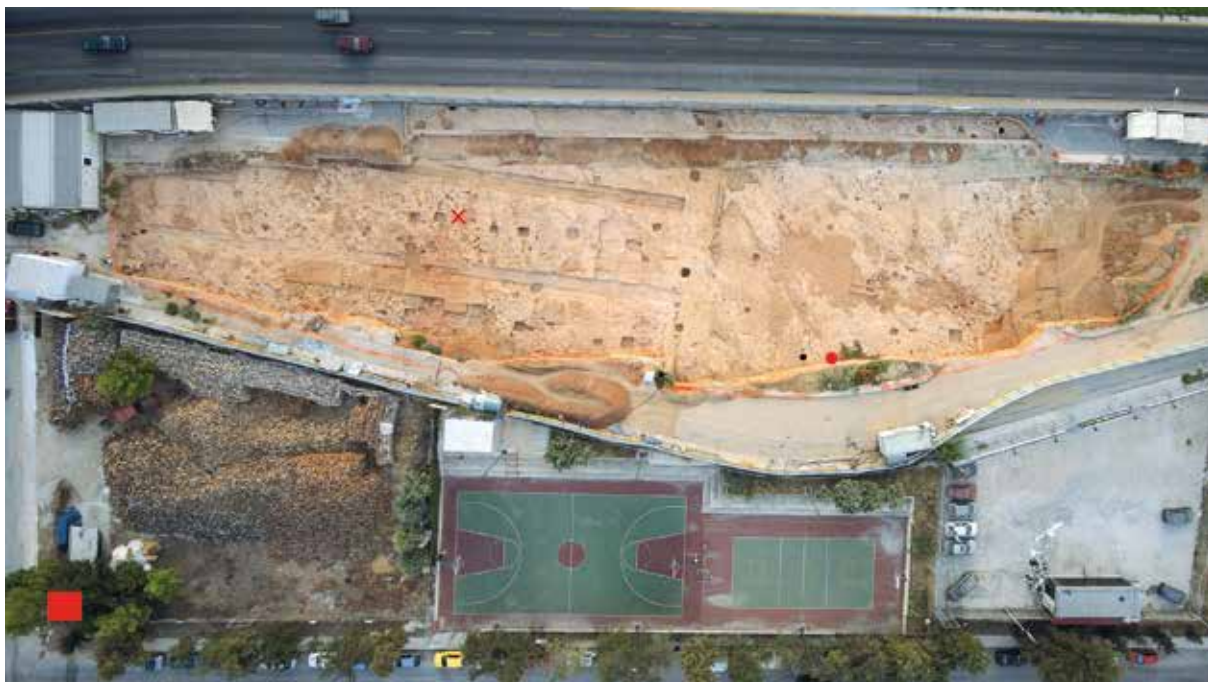
Fig. 2 The installation of Kontopigado (Building Complex III) with the location of wells 6 (●) and 7 (■) and the findspot of the figure head (X)
