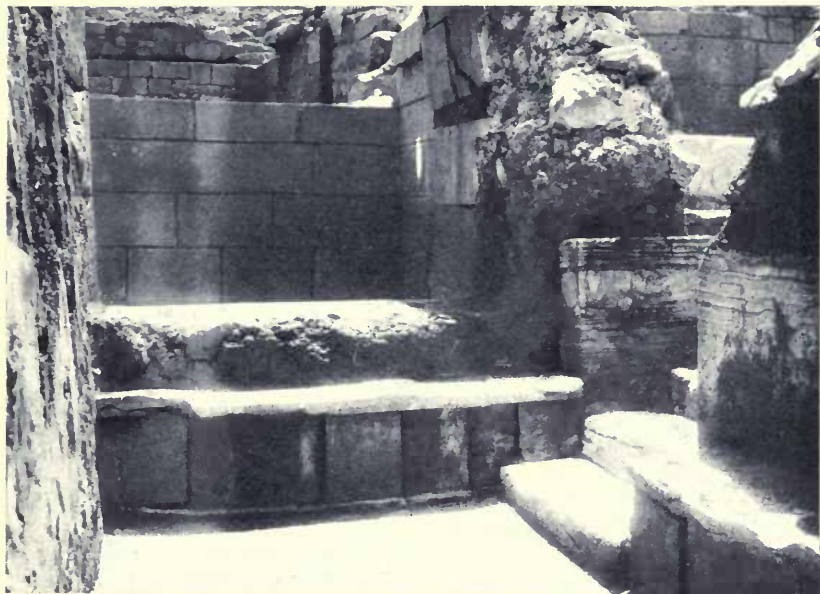
FIG. 35.—WINDOW AND SEAT WITH ALABASTER BLOCKS NEAR THE STAIRCASE IN THE VILLA OF HAGIA TRIADA.
