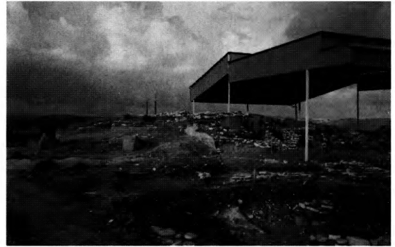
Figure 13. Kalavastos-Tenta: the site, the old shelter and the foundations for the new one.
