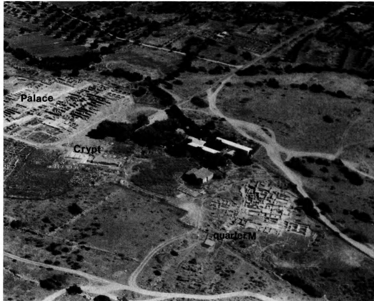
Figure 1. Mallia: aerial view from northwest, before construction of new shelters.
