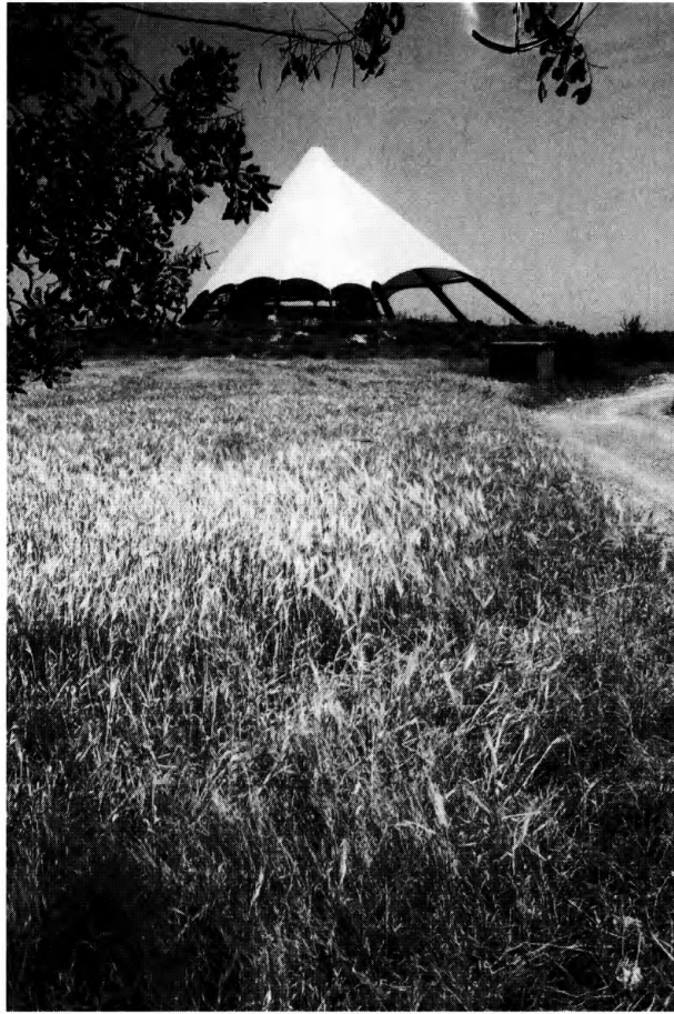
Figure 17. Kalavassos-Tenta: view of the new shelter from the north.
