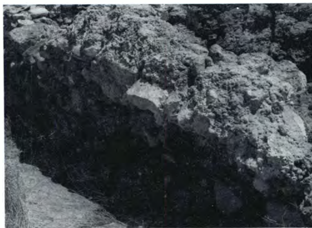
Fig. 7. Outer wall of settlement at Area 26; cement skin on upper plaster; from south-west.
