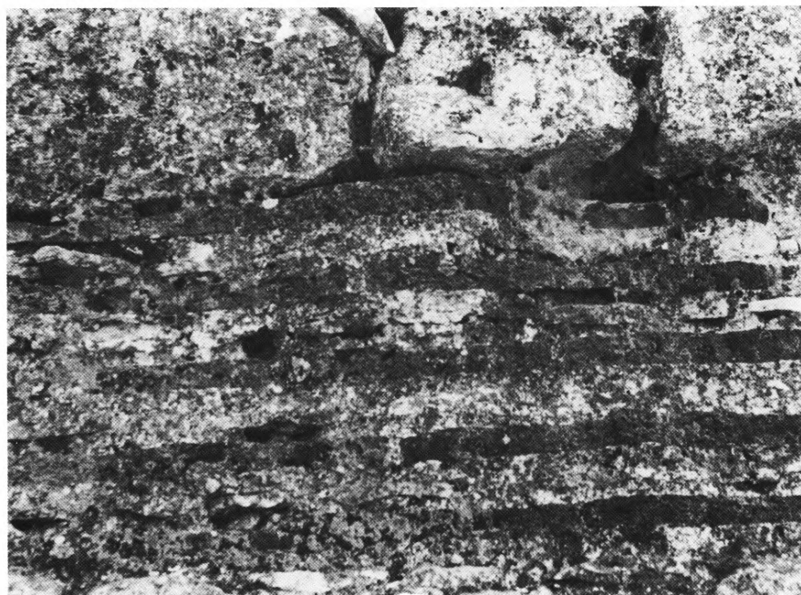
a) Ainos, Yenimahalle church. North façade, b) Midye, east gate. Intrados of arch, c) Pinarhisar. Citadel. Central tower.
