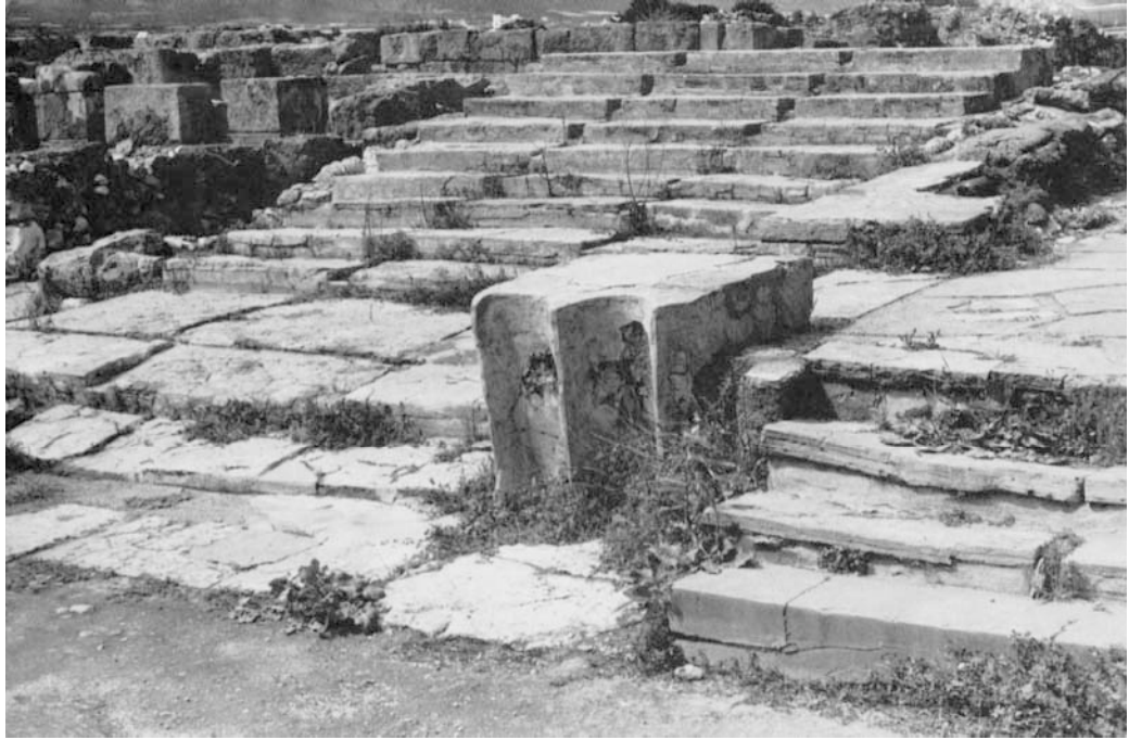
Plate 11 Mallia. Part of the east front of the West Wing, with stairs leading into area VI ( right ) and up to the first floor ( left )
