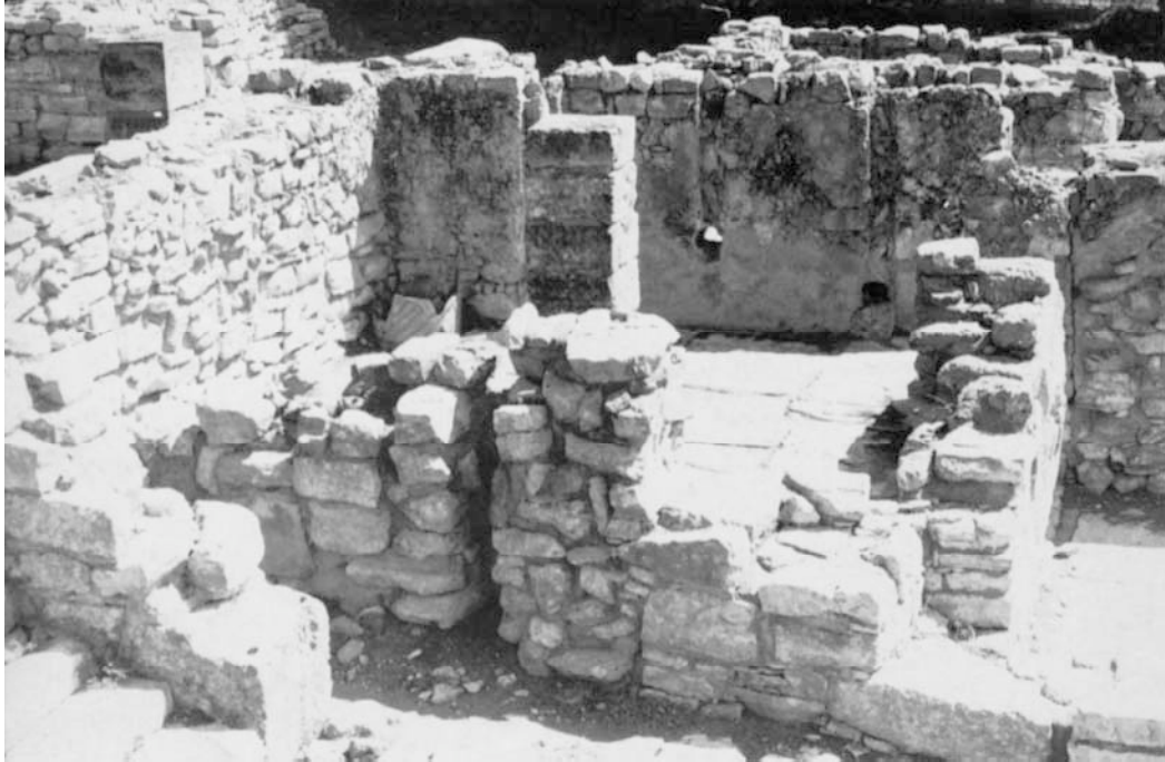
Plate 7 Tyllissos, House A, showing slots for tie-beams
