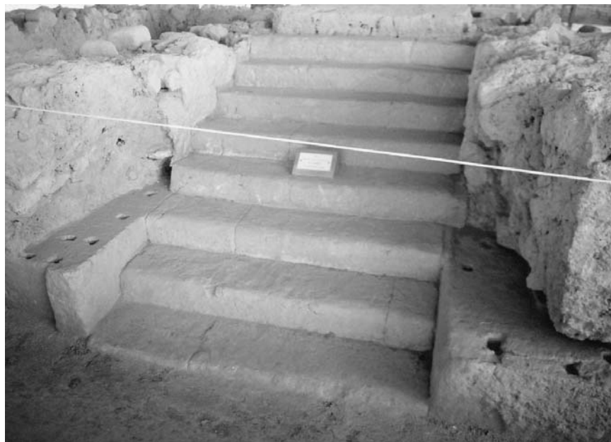
Plate 2.6 A staircase in the temple-palace at Pylos. The masonry was fixed together with bronze dowels seated in the square sockets seen on the left and right.
