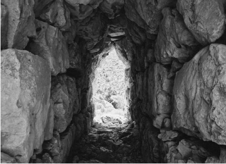
Plate 8.2 The south postern gate at Mycenae. Like Troy, Mycenae was built for siege warfare. This finely preserved tunnel through the thickness of the fortress wall was a sally-port.
