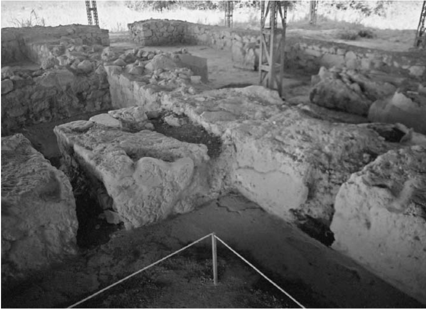
Plate 6.5 Corner of the Throne Room at Pylos, showing slots in the walls for timber framing.
